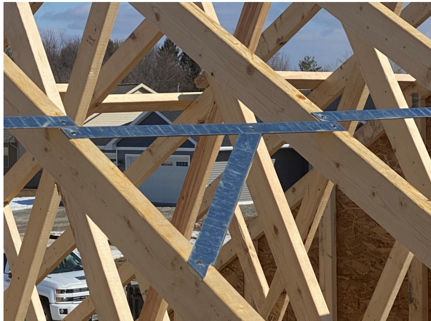
Figure 1. FastenMaster TrussBRACE Installed on Truss Top Chords
