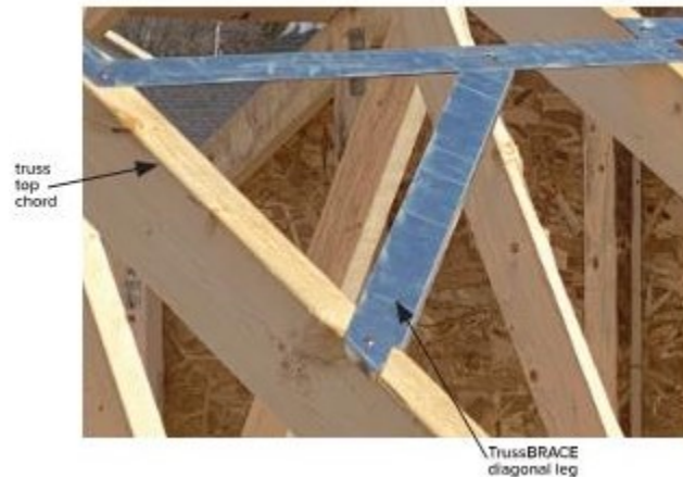
Figure 3. TrussBRACE™ Connection to Truss Top Chord
