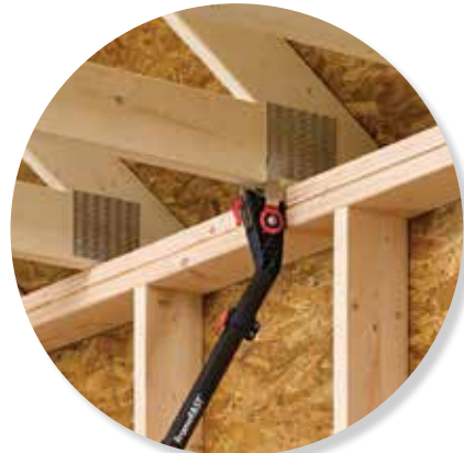
1 Truss To Top Plate
