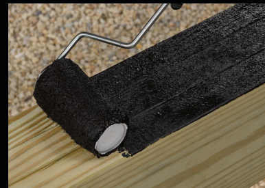
Deck Carrying Beams
